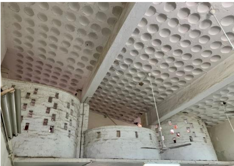
Experimentation with filler slab and brick walls at Primary Health Center at Jyoti Ltd.
